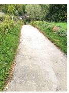
PIMLICO WAY — A firm laid hydraulically bound material from its junction with Slip Lane to the top of the rise at the end of April but either the material wasn't laid or compacted correctly or was faulty and the contractor will return
