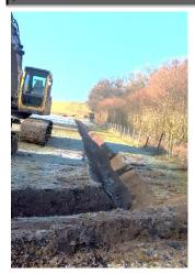
**JOHN HUGGINS** has put in a ditch/gully running alongside Slip lane (the bottom part of his field parallel to Slip Lane) which should take over 120m<sup>3</sup> of runoff water from both the fields and Pimlico. This is a cracking example of work on behalf of the community by John and whilst we know it will not actually stop any severe flooding it will slow any excess runoff from normal rainfall and therefore benefit the village. **Bev Hubbard**
