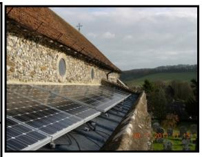
THE **SOLAR** photovoltaic (PV) system on the roof of St. Anthony's been has commissioned. The 16 panel array will produce some 3,300 kilowatt hours per year renewable electricity: about the same as that consumed by the average UK and over the 25 years
