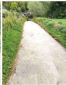
**PIMLICO WAY** – A firm laid hydraulically bound material from its junction with Slip Lane to the top of the rise at the end of April but either the material wasn't laid or compacted correctly or was faulty and the contractor will return
